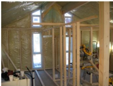
Building structure finished, Inside work on track
