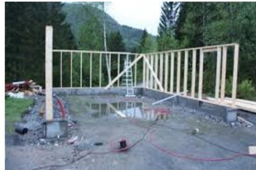
Foundation finished, building structure started
